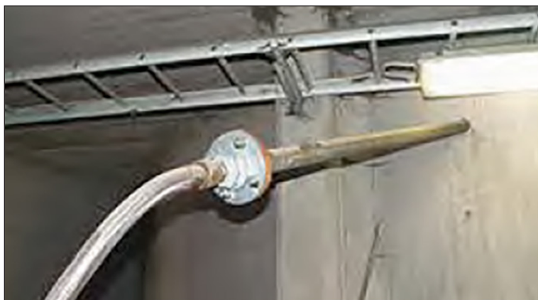
Slika 8: Sonda za ubacivanje inertnog plina. Figure 8. probe for inert gas injection (Source: Persson, Silo fires)
